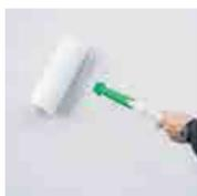
Prime the exposed render subsurface on the façade with **WP-QUARZ**. A high-grade rendering base ensures optimum adhesion and uniform drying for the subsequent layer of render. Allow façade to dry thoroughly again after priming.
